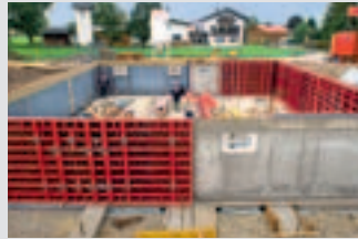
Wall Formwork
