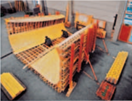
Assembly of the special elements at the Weissenhorn plant.
