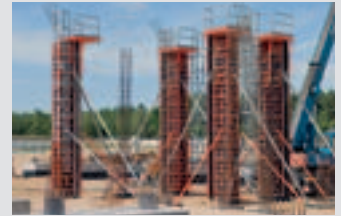
Column Formwork
