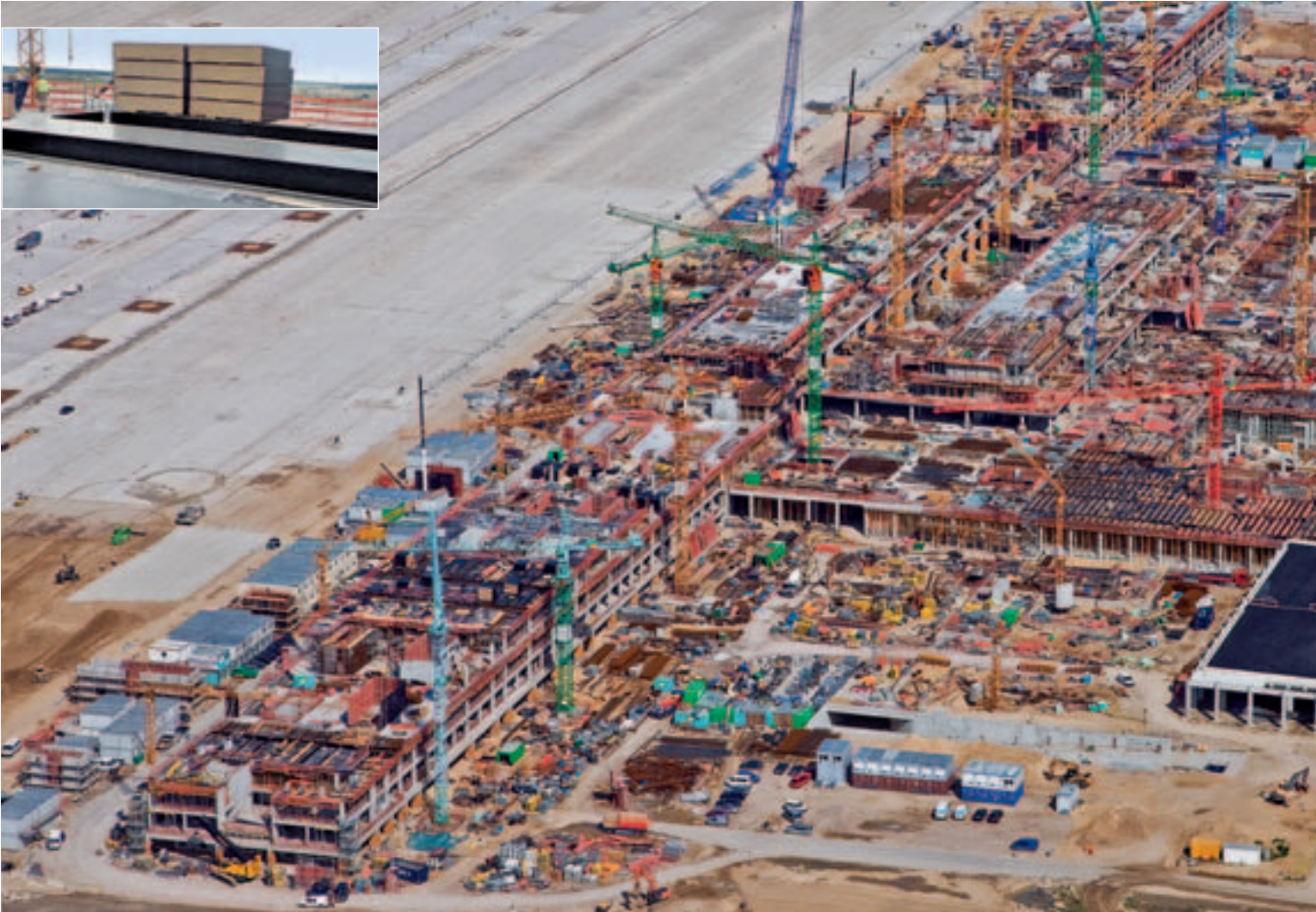
Customised slab tables for beams and box-outs for the construction of BBI Berlin Brandenburg International Airport, Berlin.
