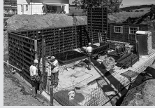
Wall Formwork
