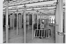
Slab Formwork
