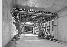
Tunnel Formwork
