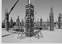
Column Formwork
