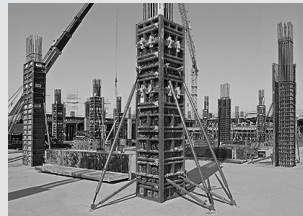
Column Formwork
