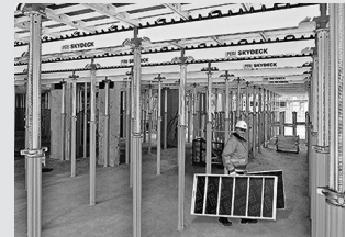
Slab Formwork
