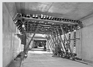
Tunnel Formwork
